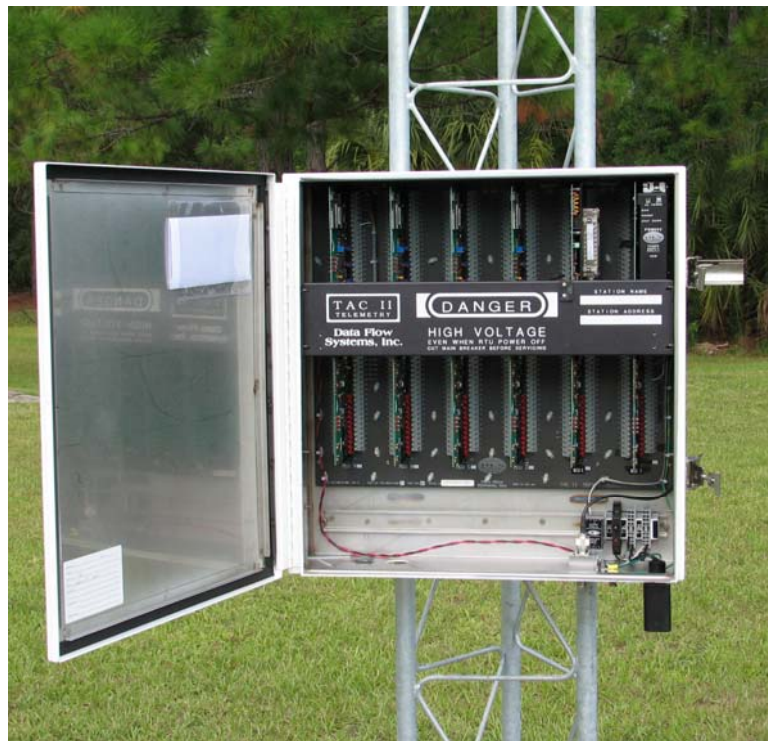
Figure 3: Modular Backplane Installed in 200 Series RTU
